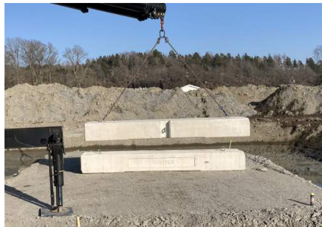
(b) Photograph from load test of working platform B.
