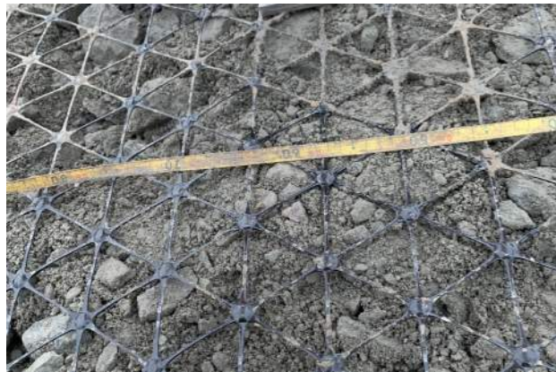
Figure 3.4: Geogrid used in field trial.
