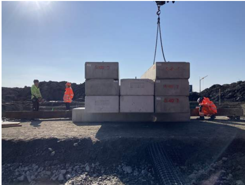
Figure 3.16: Photograph of test G as it is fully loaded.
