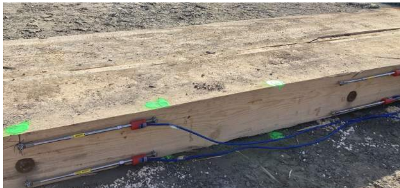
(a) Crackmeters installed on a log mat.
